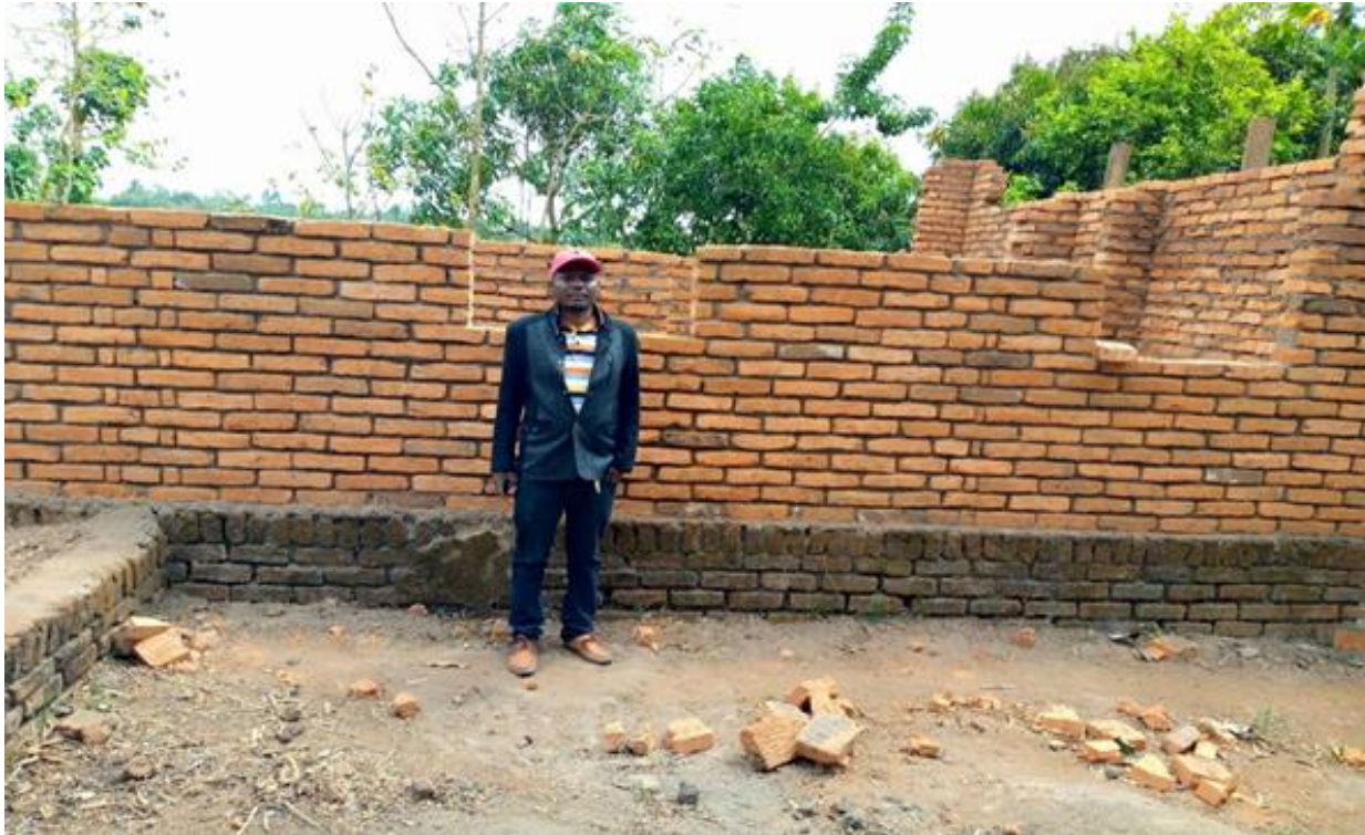
Photo 4 : New house for Kalepa's is underway
